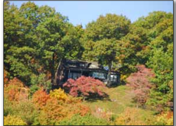
Natural building materials, earthtone colors, and intact vegetative screening make this home appear to blend into the hillside.
