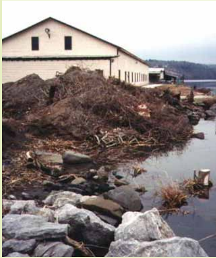
Shoreline before restoration.
