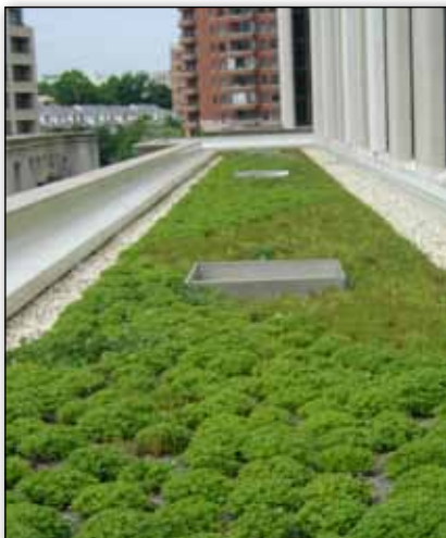
Vegetated green roofs save energy and reduce stormwater run-off.
