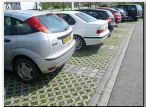
Permeable paving of parking swales.
