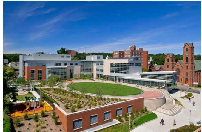
SUNY-Orange, Newburgh Campus vegetated roof and rainwater harvesting system (Image courtesy of SUNY-Orange)
